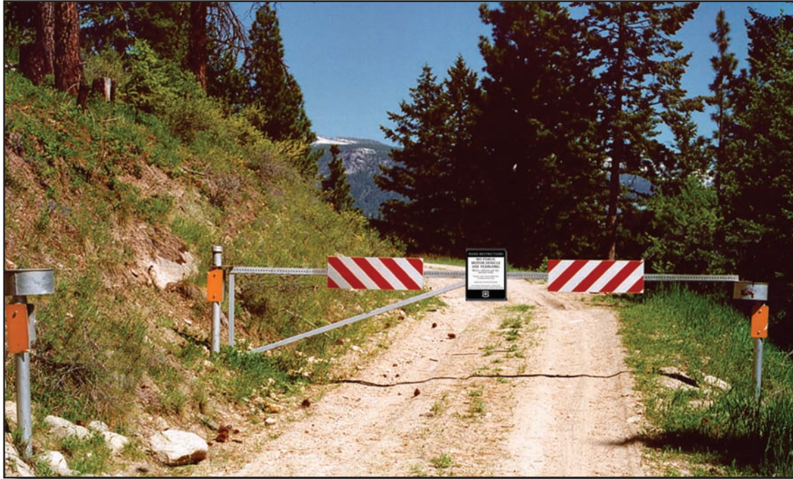
Figure 23—Maintenance level 2 single-lane road with native surfacing that has motor vehicle use restricted by a gate. The surface and shoulders of this maintenance level 2 road are adequate for access by high-clearance vehicles at low speeds, and there is no evidence of significant environmental damage. A gate is an appropriate closure device for maintenance level 2 roads that temporarily restrict all motor vehicle use or that are managed as administrative use only roads. If motorized or nonmotorized use, such as bicycles, occurs behind a gate, the back side may require signing also.
