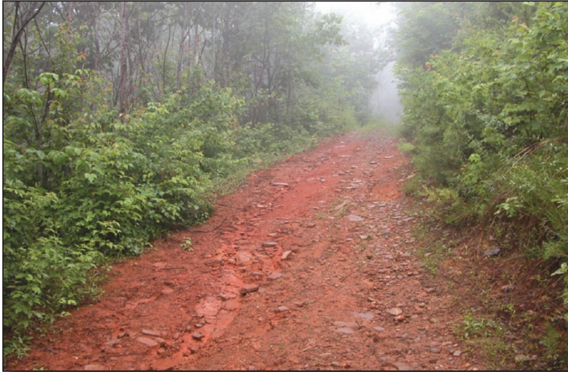
Figure 18—Maintenance level 2 single-lane road with pit-run surface. This road is currently passable by high-clearance vehicles at low speeds and there is no evidence of significant erosion. No immediate maintenance is needed and future surface and shoulder maintenance activities should be limited to maintaining passage by high-clearance vehicles and to keep drainage features functional.
