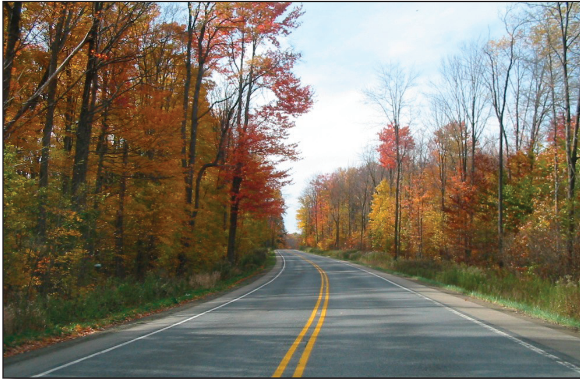
Figure 4—Maintenance level 5 double-lane road with no-passing zone and edge markings, an asphalt surface, and asphalt shoulders. The road is free of litter and the maintenance of the roadside vegetation provides adequate sight distance. Remove danger trees as required. It is acceptable to mark a double-lane road entirely with no-passing zone markings as shown in the photo.
