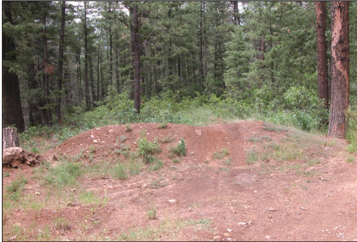
Figure 24—Maintenance level 1 road that has been blocked to motor vehicles by an earth mound. Design closure features to avoid creating hidden hazards to users, such as snowmobilers and bicyclists. An example of a hidden hazard is deep trenching behind the earth mound.
