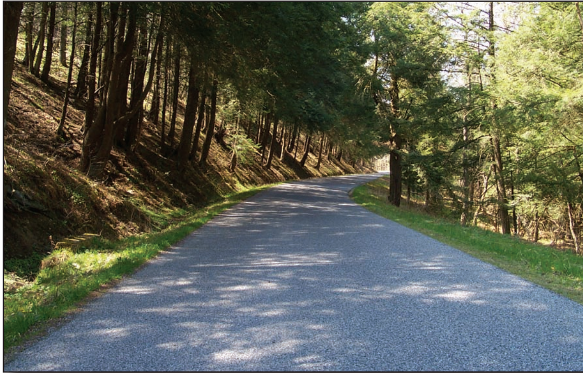
Figure 7—Maintenance level 4 double-lane road with a chip-seal surface and no shoulders. Ditches are kept clean to facilitate drainage. The road is free of litter, and the maintenance of the roadside vegetation provides adequate sight distance. Centerline and edge markings are not required on double-lane paved nonurban roads. Curves and other hazards should be marked with warning signs if advised by a documented engineering judgment or engineering study.
