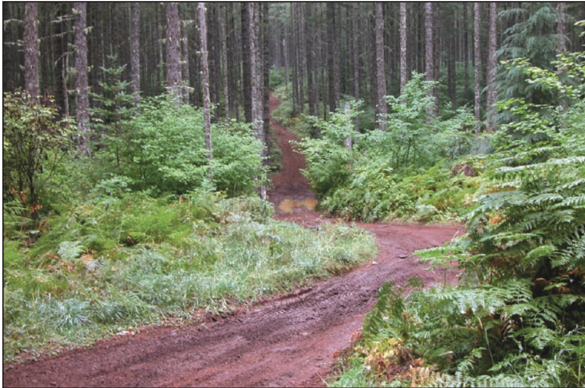
Figure 19—Maintenance level 2 single-lane road with native surface. This road is passable by high-clearance vehicles at low speeds even though some rutting of the traveled way is evident. Rutting on the road surface should be corrected at the next scheduled maintenance if it begins to cause unacceptable environmental damage.
