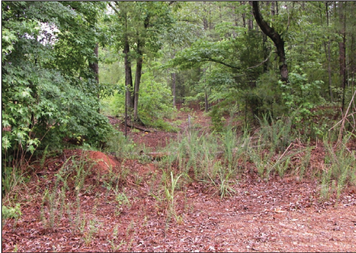
Figure 29—Maintenance level 1 road with motor vehicles eliminated by a vegetated earth mound, which both disguises and physically blocks the road.
