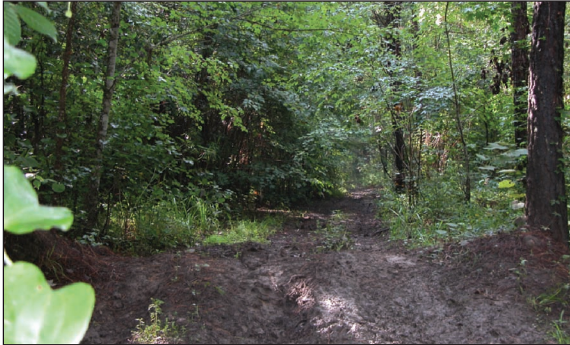
Figure 22—Maintenance level 2 single-lane road with native surface. This road surface is passable by high-clearance vehicles at low speeds and does not require surface maintenance unless significant erosion is occurring. Rutting on the road surface should be corrected at the next scheduled maintenance if it begins to cause unacceptable environmental damage. There is significant vegetation encroachment that could make the road impassable. The encroaching vegetation should be logged out and brushed to provide passage by high-clearance vehicles.
