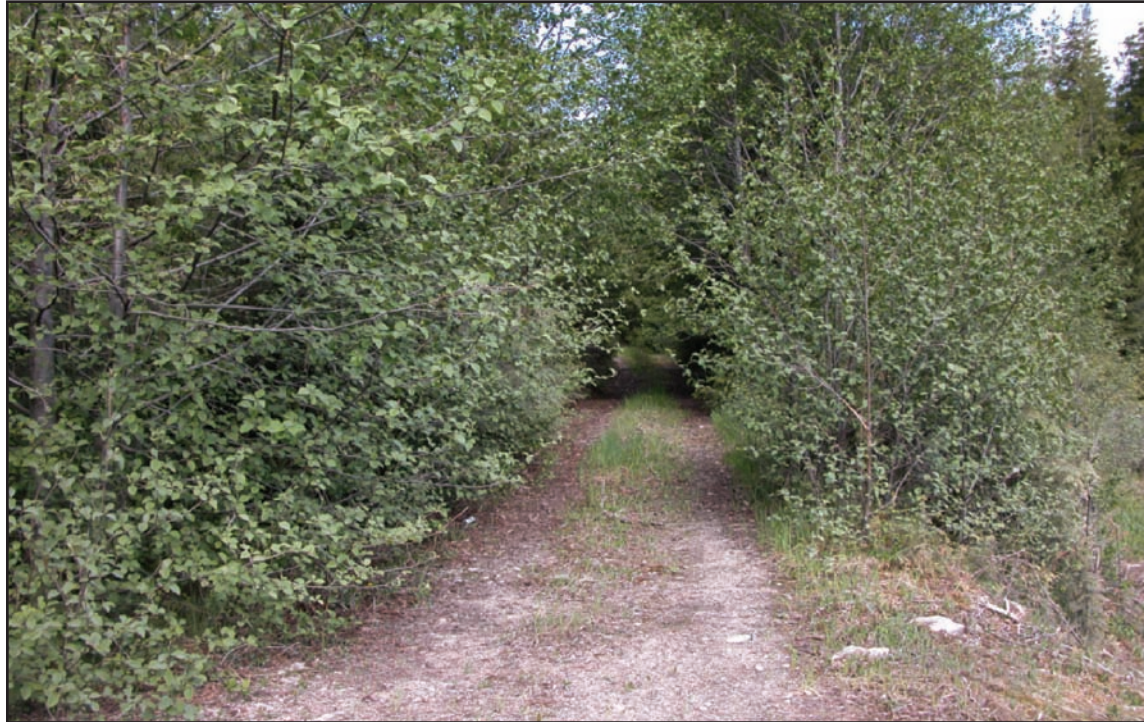
Figure 20—Maintenance level 2 single-lane road with pit-run surface. The surface on this road is maintained adequately for high-clearance vehicles at low speed, and there is no evidence of erosion. However, the vegetation on the shoulder is beginning to encroach onto the traveled way and should be maintained to allow for access by high-clearance vehicles and maintenance equipment. The grass growing on the road surface is acceptable since it is not affecting passage.
