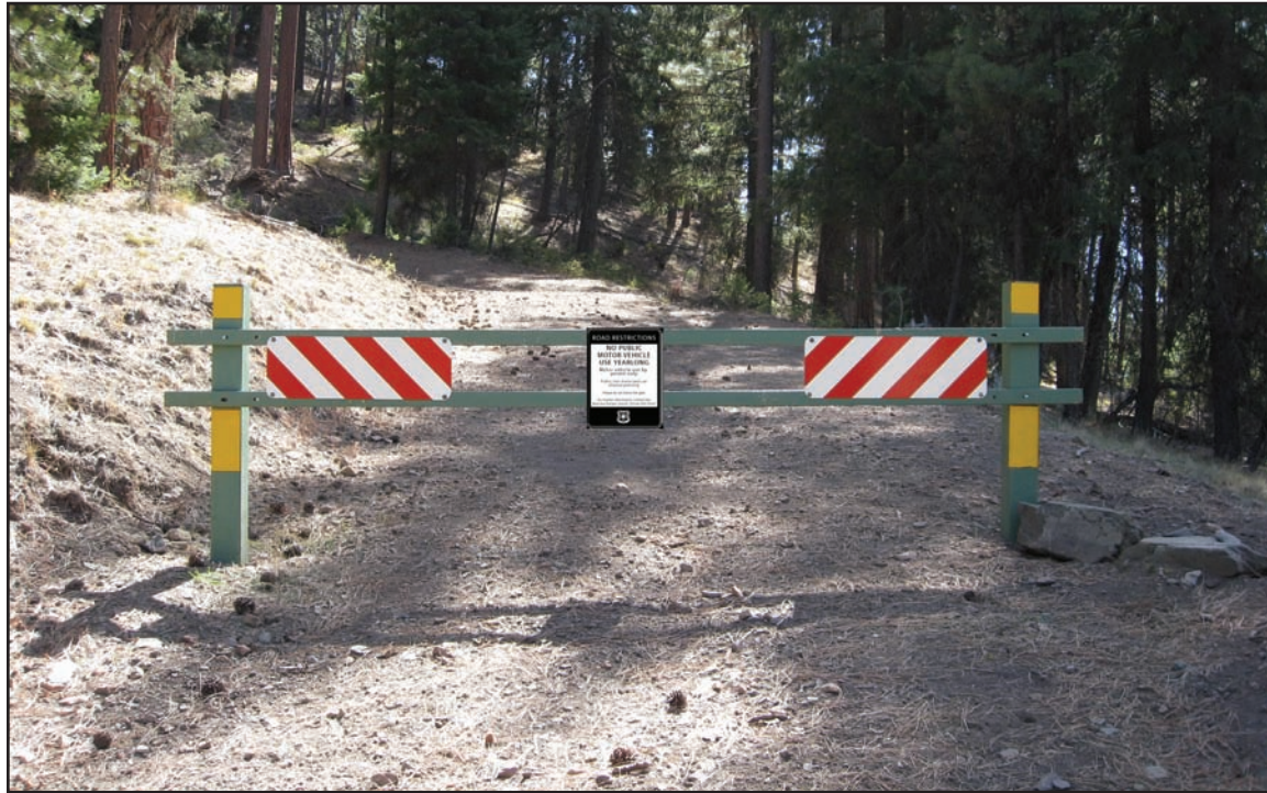
Figure 30 - Maintenance level 1 road with motor vehicle use restricted by a barricade. The road is closed to all motor vehicle use, including administrative use, for a period of more than 1 year. Gates are not appropriate on level 1 roads. Appropriate travel management signs may be placed on the barricade to display restrictions and/or reasons for closures. If motorized or nonmotorized use, such as bicycles, occurs behind a barrier, the back side also will require signing.
