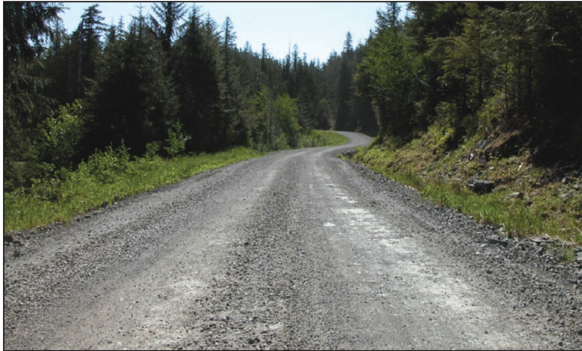
Figure 13—Maintenance level 3 single-lane road with a gravel surface and gravel shoulders. Maintain the crown and keep the drainage functional by properly maintaining the ditches. In the road shown above, removing the berms from the road edge and removing vegetation and other material that would impede the flow of water off the road and through the ditch would improve the drainage. The road is free of litter and the maintenance of the roadside vegetation provides adequate sight distance. Curves and other hazards should be marked with warning signs if advised by a documented engineering judgment or engineering study.
