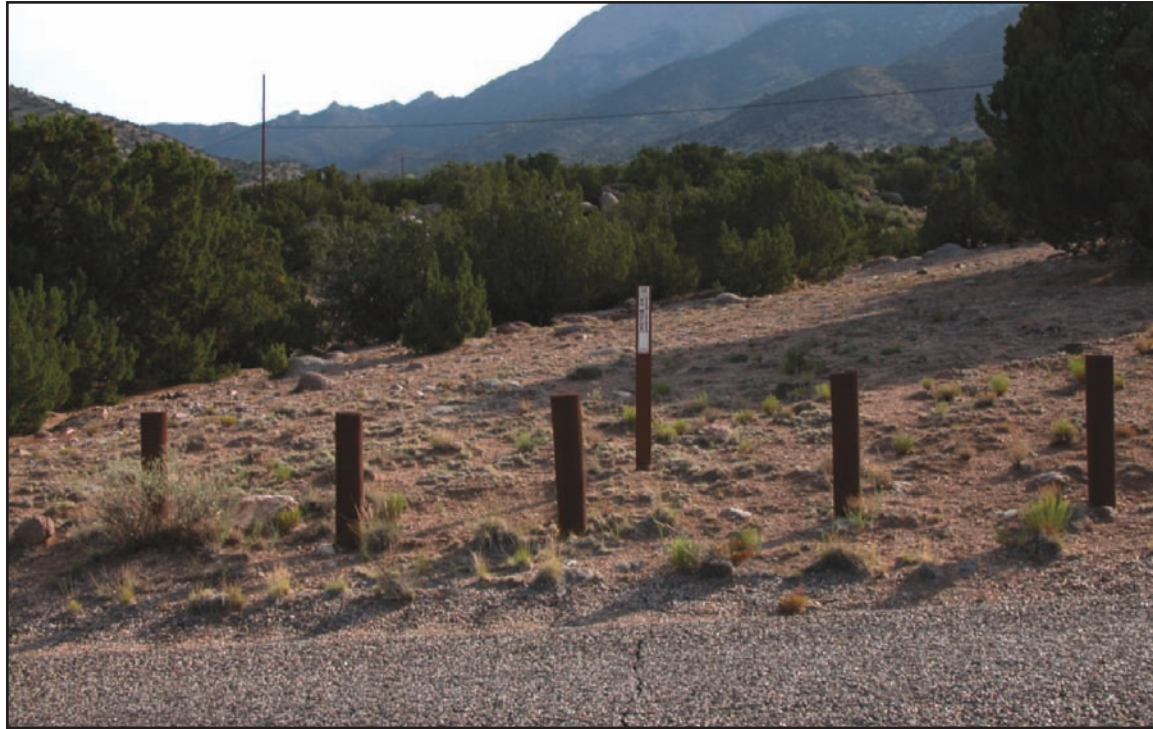
Figure 27—Maintenance level 1 road that has been blocked to highway vehicle traffic by posts and includes a sign prohibiting motorized vehicles. Use type 2 object markers if the posts present a hazard. Wooden posts are easily cut or damaged and removed and may not be an effective closure. Use posts in areas that are patrolled on a regular basis, or near high-use areas. Road restricted signs, with or without reasons, may be used. Route numbers should be displayed on a separate vertical marker from the restriction sign.
