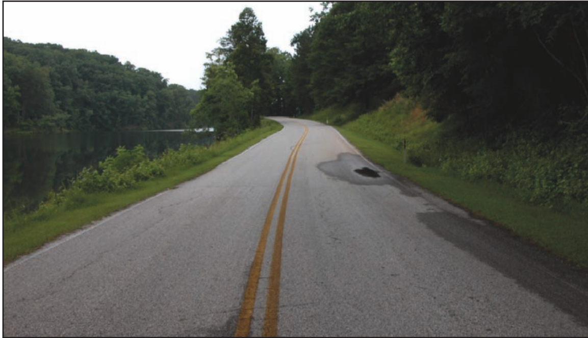
Figure 2—Maintenance level 5 double-lane road with no-passing zone markings, an asphalt surface, and unpaved shoulders. Grass on shoulders is acceptable and helps with stabilization. Leaving vegetation that does not interfere with sight distance helps stabilize the backslope. As potholes and depressions begin to develop they should be corrected to continue providing a high degree of user comfort and convenience. Curves and other hazards should be marked with warning signs if advised by a documented engineering judgment or engineering study. It is acceptable to mark a double-lane road entirely with no-passing zone markings as shown in the photo.
