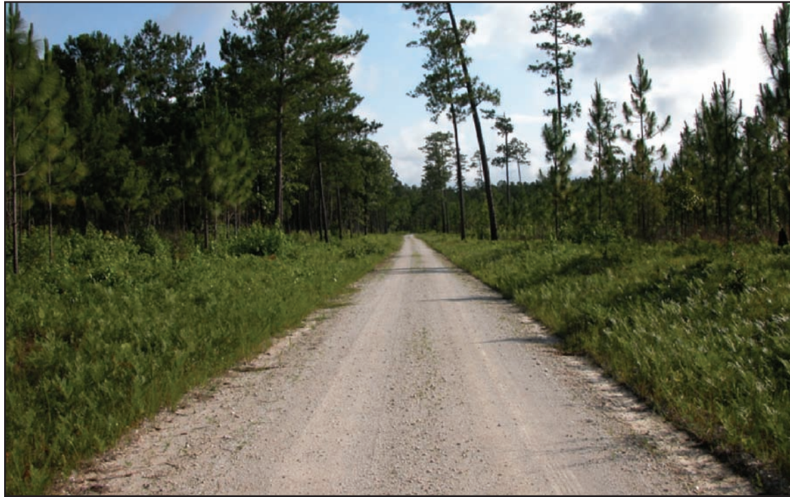
Figure 12—Maintenance level 3 single-lane road with a gravel surface and gravel shoulders. Road surface should be maintained to provide adequate drainage and to provide for travel by prudent drivers in standard passenger cars and not to increase the user comfort and convenience above that expected for a maintenance level 3 road. User comfort and convenience are not considered priorities. The base course and surfacing should be replaced as needed to protect the resource.
