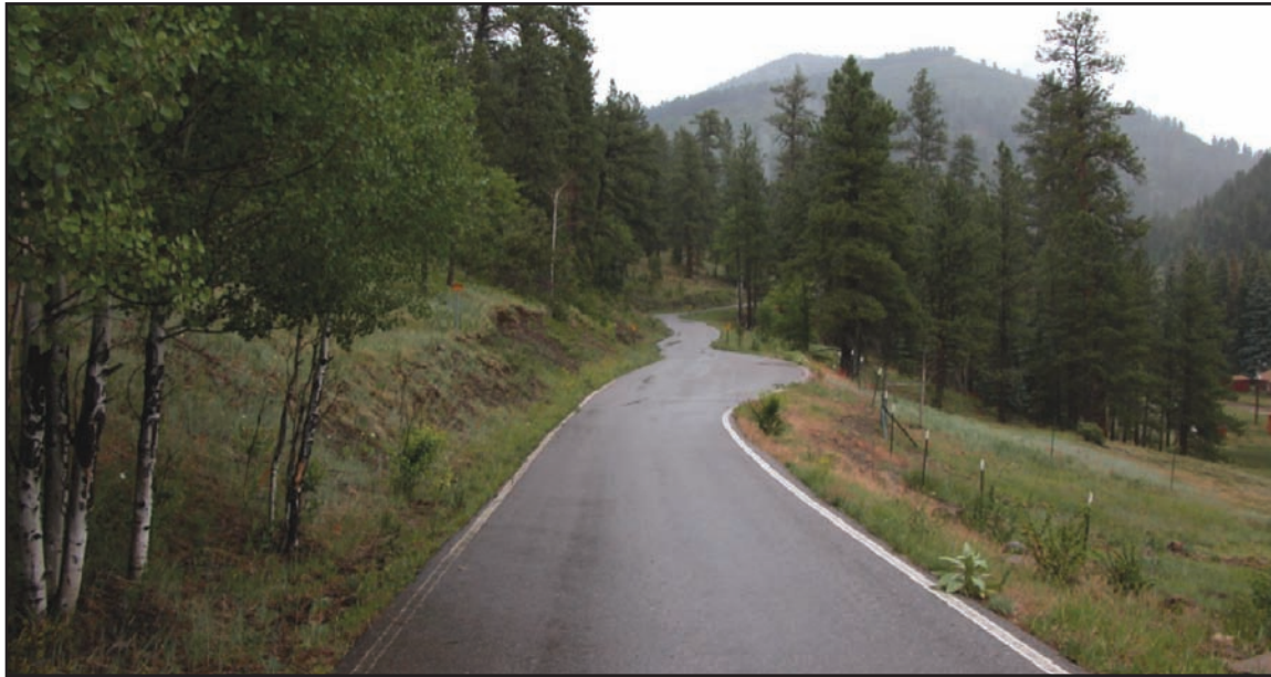
Figure 8—Maintenance level 4 single-lane road with asphalt surface, no shoulders, paved turnouts, and edge markings. It may be desirable to place edge markings when the road has narrow lanes and shoulders as shown in the photo. If it has been determined that edge markings are necessary they should be maintained appropriately. A broken white lane line, with entry and departure breaks, may be used at turnouts to provide continuity of guidance and define the turnout lane. If pavement width is less than required for the travel lane and turnout, mark an uninterrupted uniform lane width without identifying a turnout. The road is free of litter and the maintenance of the roadside vegetation provides adequate sight distance. Curves and other hazards should be marked with warning signs if advised by a documented engineering judgment or engineering study.
