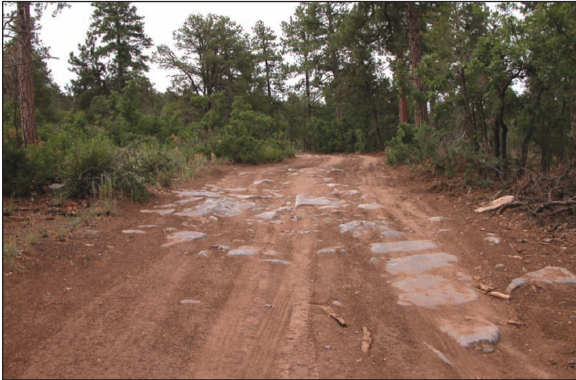
Figure 21—Maintenance level 2 single-lane road with native surface. While the surface on this road is extremely rough, it is still passable by high-clearance vehicles at low speeds. Generally, no additional surface maintenance is required unless unacceptable environmental damage due to erosion or widening occurs.
