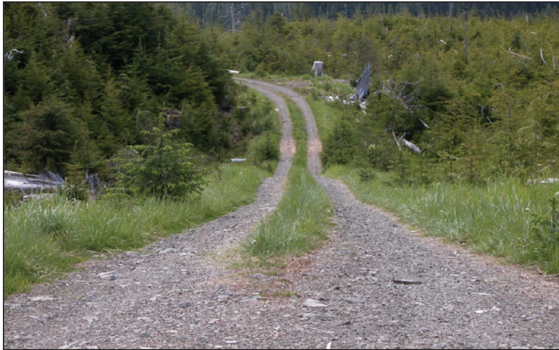
Figure 17—Maintenance level 3 single-lane road with a gravel surface and no shoulders. Maintain road surface to provide adequate drainage. Surface roughness is acceptable if maintained for travel by a prudent driver in a standard passenger car. Remove berms and vegetation from the middle of the road that would impede travel by a prudent driver in a standard passenger car. Maintain drainage facilities, such as culverts and drainage pipes, so they are functional and prevent unacceptable environmental and resource damage.
