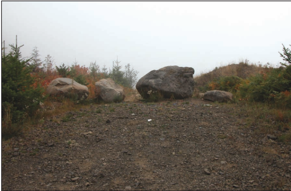
Figure 26—Maintenance level 1 road that has been blocked to motor vehicles by boulders. Partially bury boulders and arrange them in a nonlinear pattern for a more natural look. Boulders may not be an effective natural barrier if adjacent vegetation is grass and light brush. Vertical route markers may be used but are not prominently displayed.
