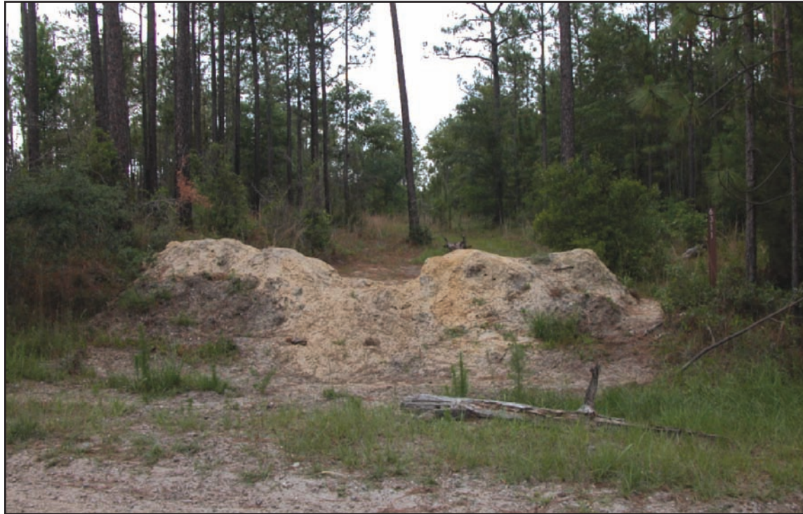
Figure 25—Maintenance level 1 road that has been blocked to motor vehicle traffic by an earth mound. Constructing a berm in a relatively flat terrain (i.e., minimal cut and fill) is a challenge. Periodic maintenance of the closure may be needed to ensure that it is an effective closure. Design the closure features to avoid creating hidden hazards to users, such as snowmobilers and bicyclists. An example of a hidden hazard is deep trenching behind the earth mound.
