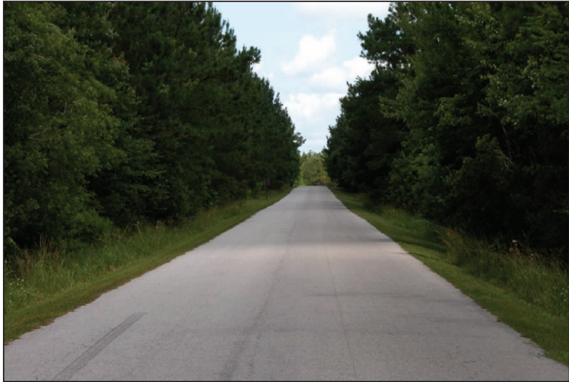
Figure 5—Maintenance level 5 double-lane road with no centerline, no edge marking, a chip-seal surface, and unpaved shoulders. Grass on shoulders is acceptable and helps with stabilization. It is acceptable not to place centerline and/or edge markings on a double-lane nonurban road.
