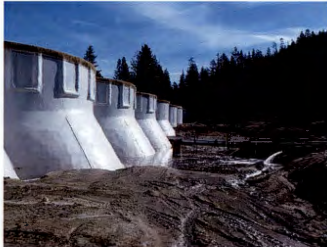
Hume Lake Dam, Sequoia National Forest, California.
