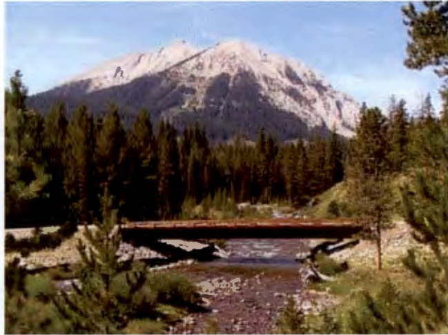
Taylor Fork Bridge, Gallatin National Forest, Montana
